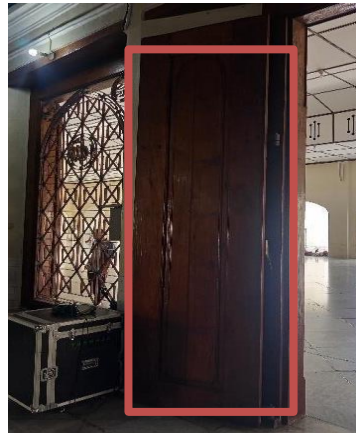
Figure 15. Main Mosque Door
