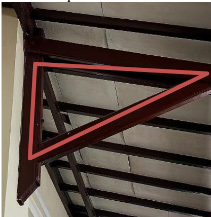
Figure 13. Mosque Roof Supports
