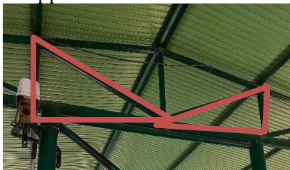
Figure 12. Parking Roof Supports
