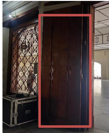
Figure 15. Main Mosque Door
